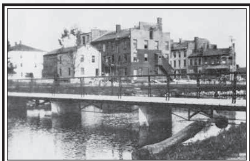
FROM A FOOTBRIDGE OVER THE OLD MILLRACE ABOUT 1910, YOU SEE THE FORMER WASHTENAW HOUSE HOTEL AT LEFT, THE BACK OF THE THREE-STORY ANSON BROWN BUILDING, CENTER, AND THE HURON BLOCK ACROSS BROADWAY, RIGHT.
